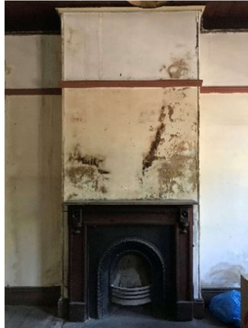
Figure 55 - First floor fireplace and surround, including retained firebox. Note the water damage across the chimney breast, presumably from the chimney above.
