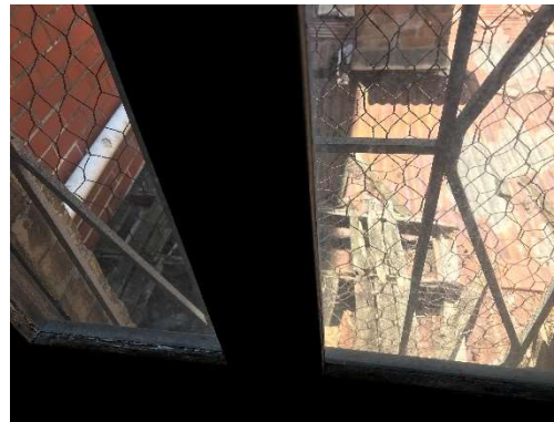
Figure 57 - View through the door shown in Figure 56 showing the remnant collapsed timber structure of the former balcony.
