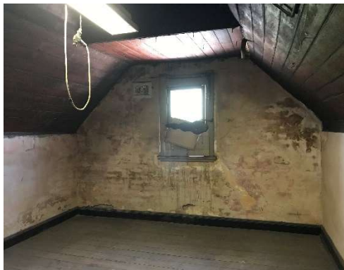
Figure 60 - Second floor - view towards the window facing the Pacific Highway. Note the level of water damage to the internal plasterwork.
