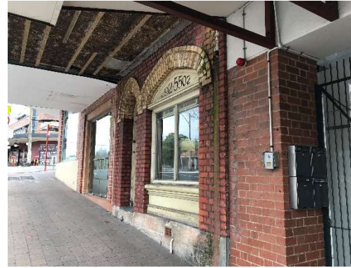
Figure 35 - An alternative view of the facade which includes the soffit of the awning. The soffit is in very poor condition; with this image also showing the water damage to the façade and the poor condition of the joinery.
