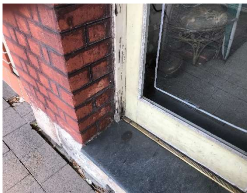
Figure 38 - The slate door threshold, with damage to the timber door frame evident. Note the tuckpointing the brickwork.
