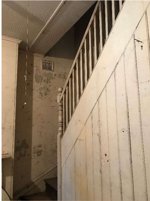
Figure 44 - Commencement of the staircase from ground floor. The first set of timber winders have deteriorated and require reconstruction. This stair is also non-compliant in a number of ways.
