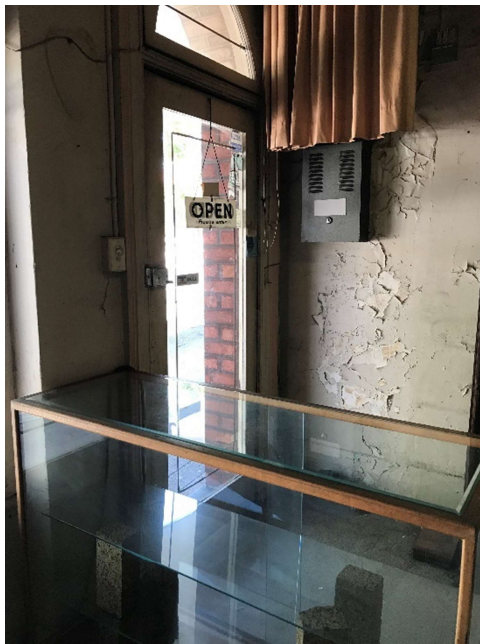
Figure 42 - Evidence of water entry in the ground floor shop space.
